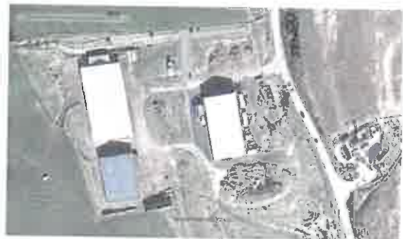
Figure 5: 2009 Aerial image (Google Earth)
